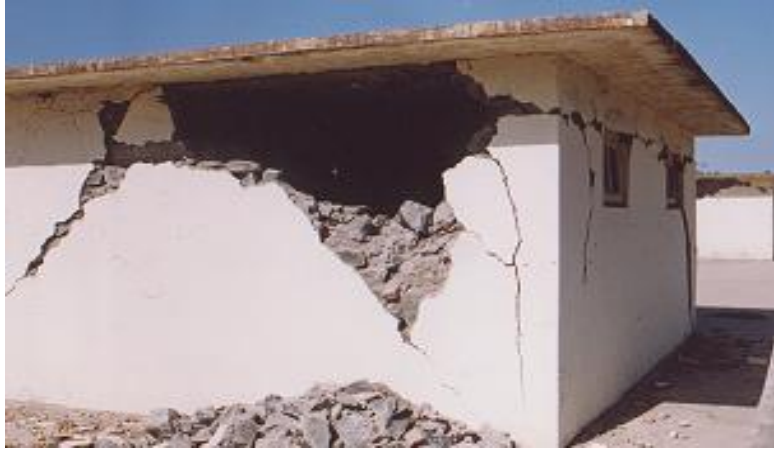
Plate 6: Separation of roof from walls
