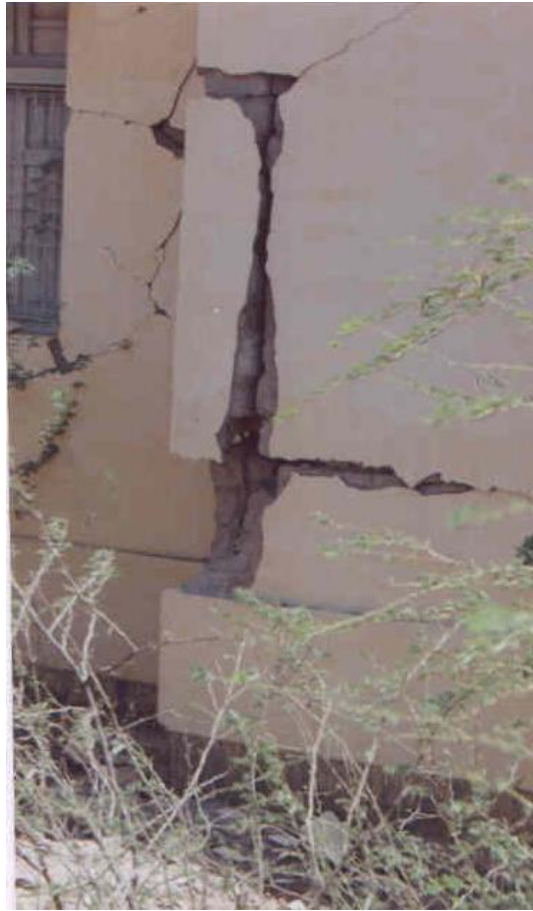
Plate 2: Separation of wall at junctions
