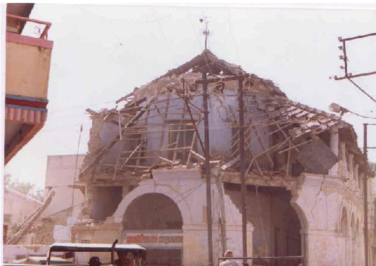
Plate 1: Out-of-plane flexure failure
