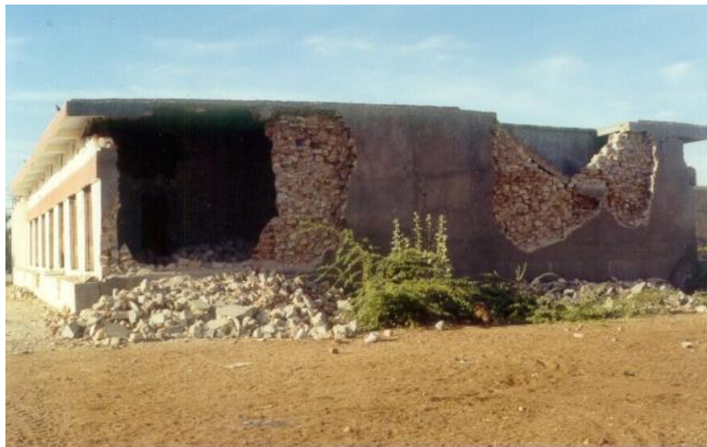
Plate 5: Buckling of wythes
